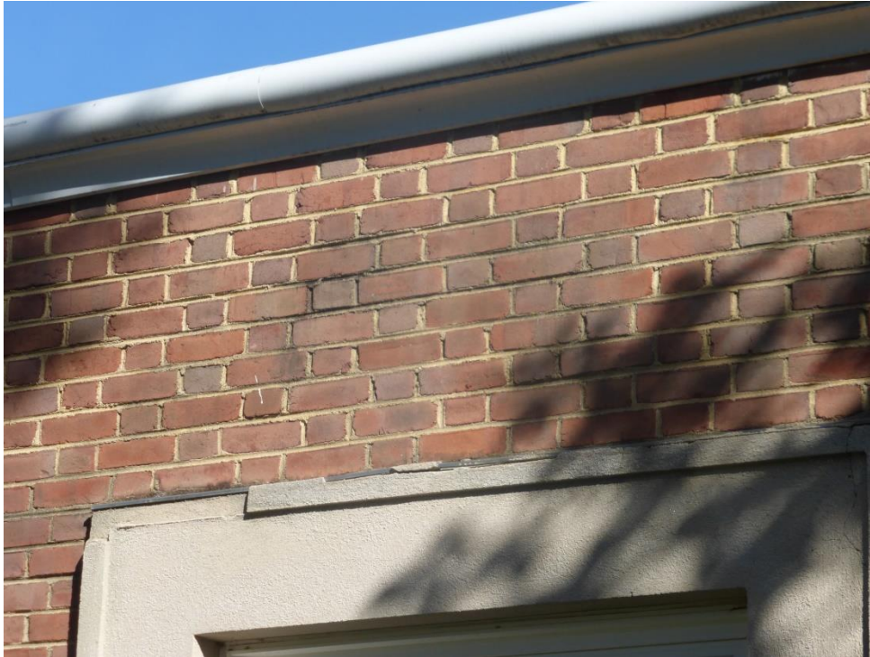
Spalling of Precast Window Trim from Water Infiltration
