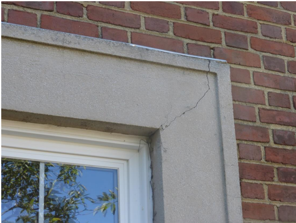
Cracking of Precast Window Trim Occurs at Most Windows
