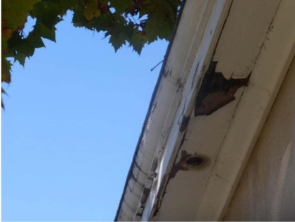
Damage to Soffit Overhang from Leaking Built In Gutter
