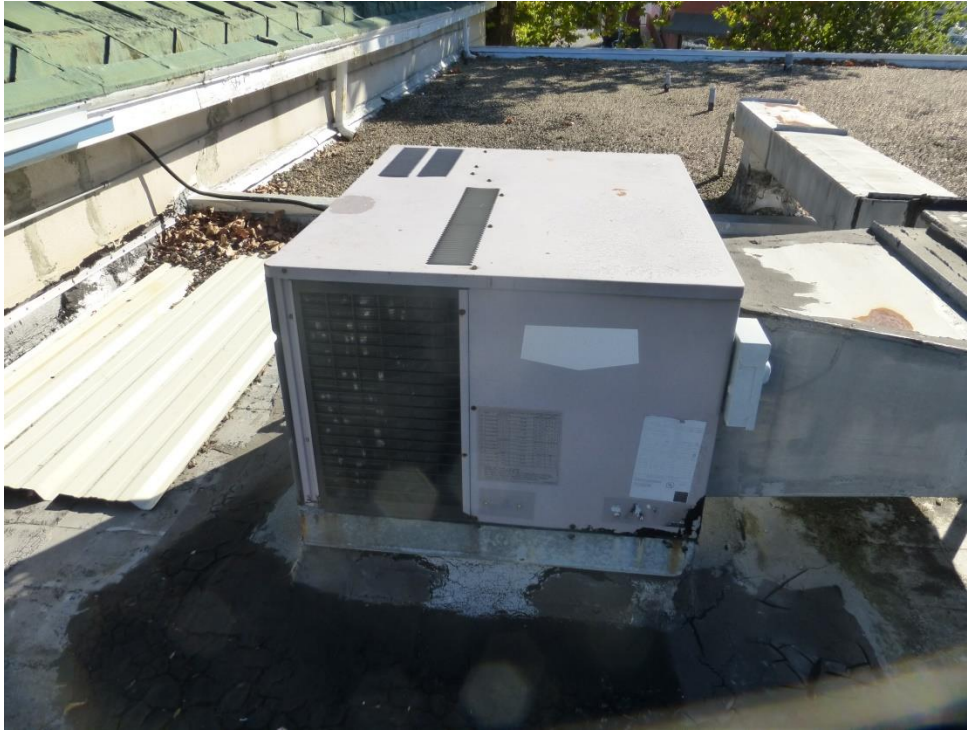
HVAC Unit and Associated Ductwork on Flat Roof Addition
