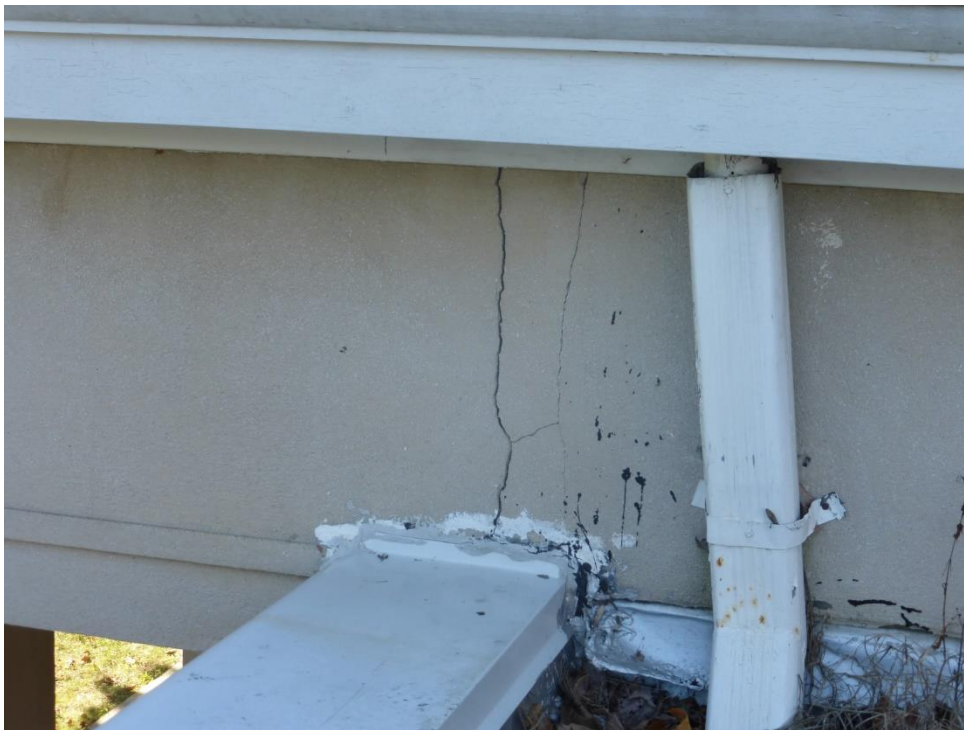
Cracks Common in Stucco Band Below Built In Gutter
