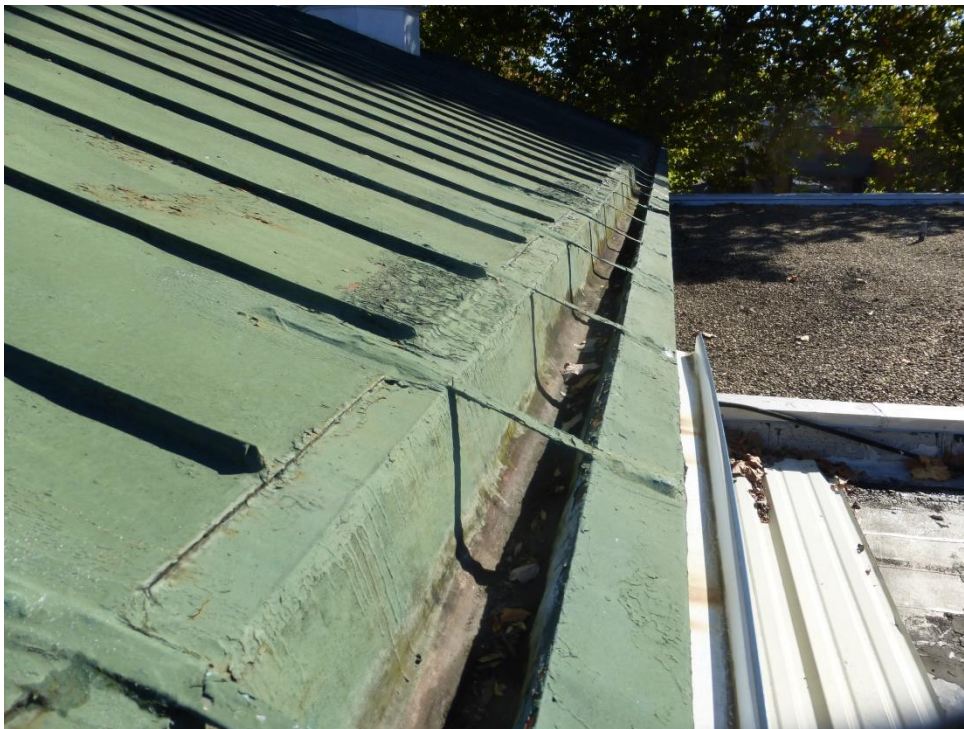
Built In Eave Gutter in Standing Seam (Tin Roofing)
