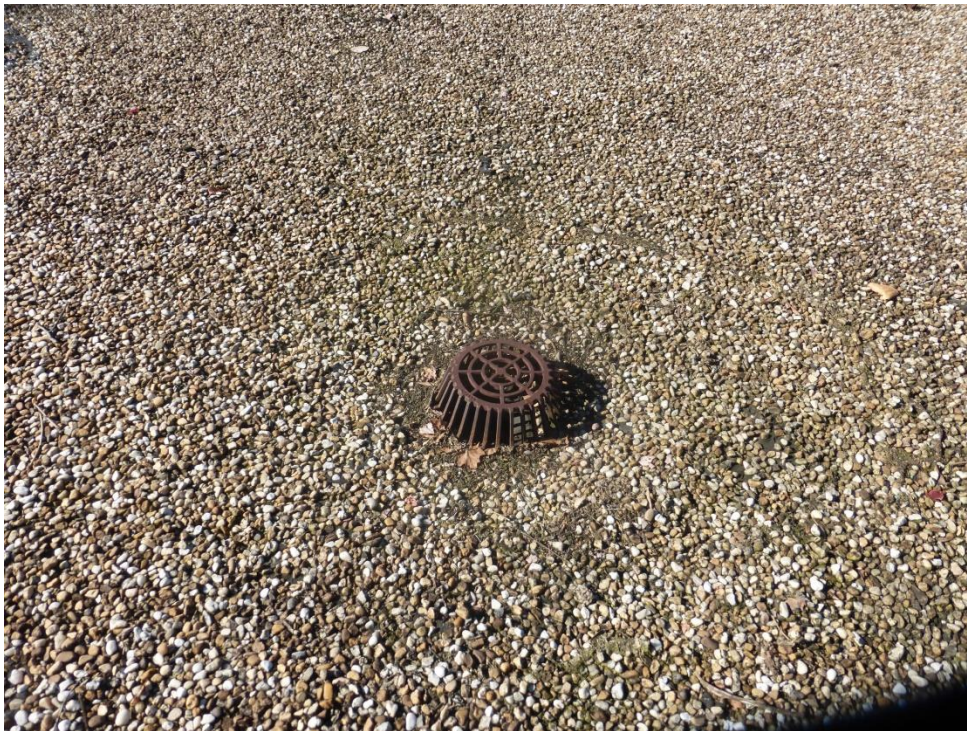
Typical Roof Drain- One of Two
