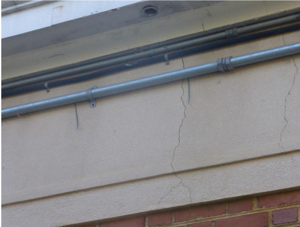
Cracks in Stucco Band Below Built In Gutter
