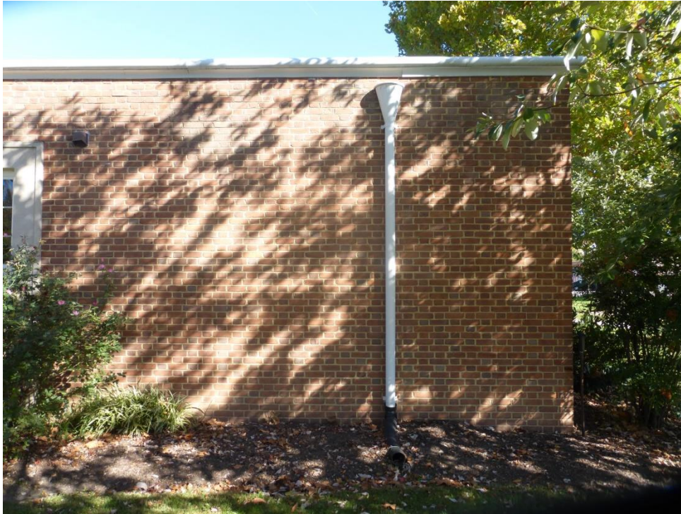
Typical Conductor Head and Down Spout
