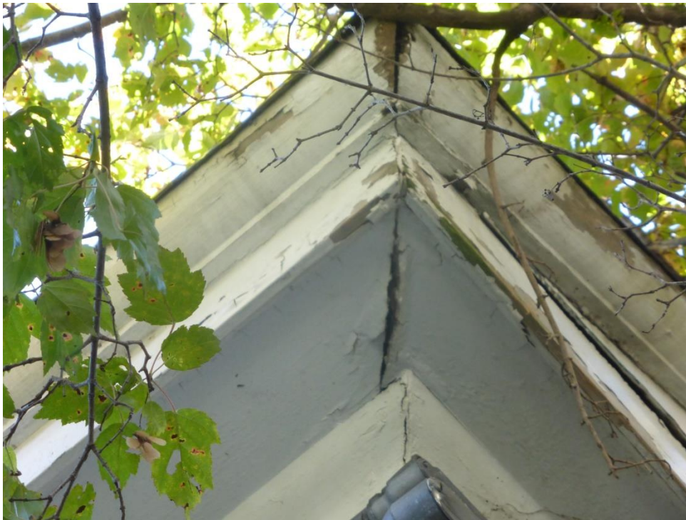
Damage to Soffit Trim from Leaks in Built In Gutter
