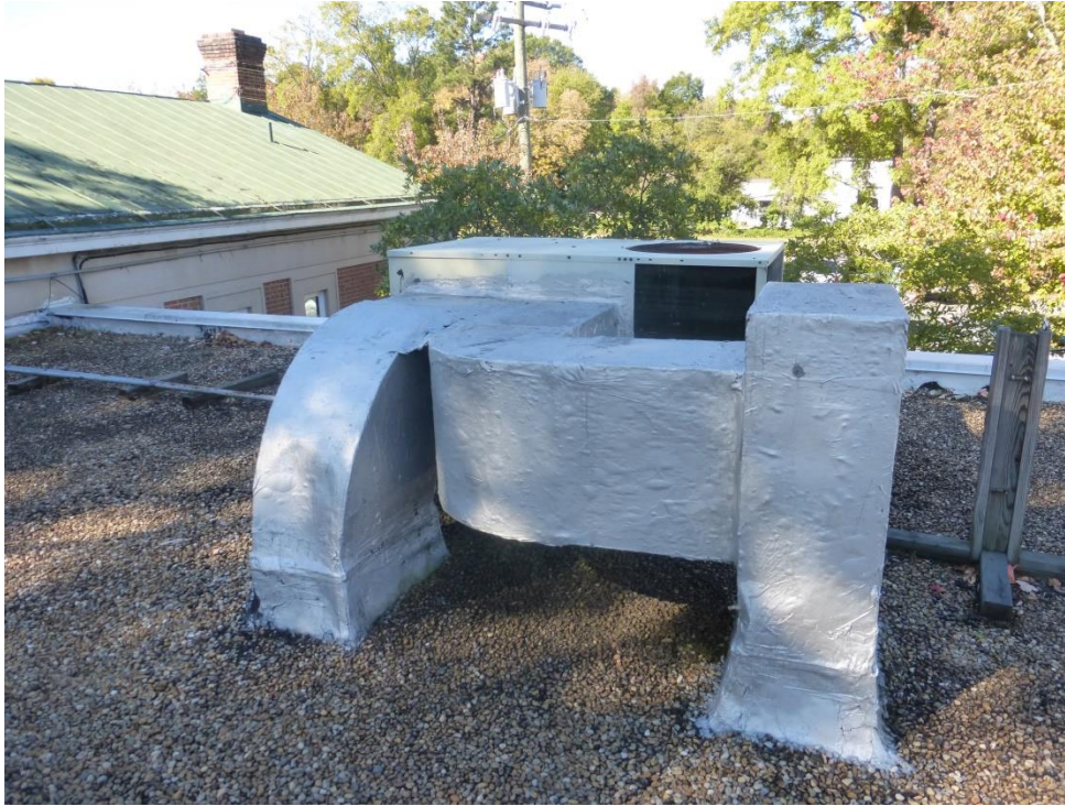
HVAC Unit and Associated Ductwork on Original Flat Roof Area
