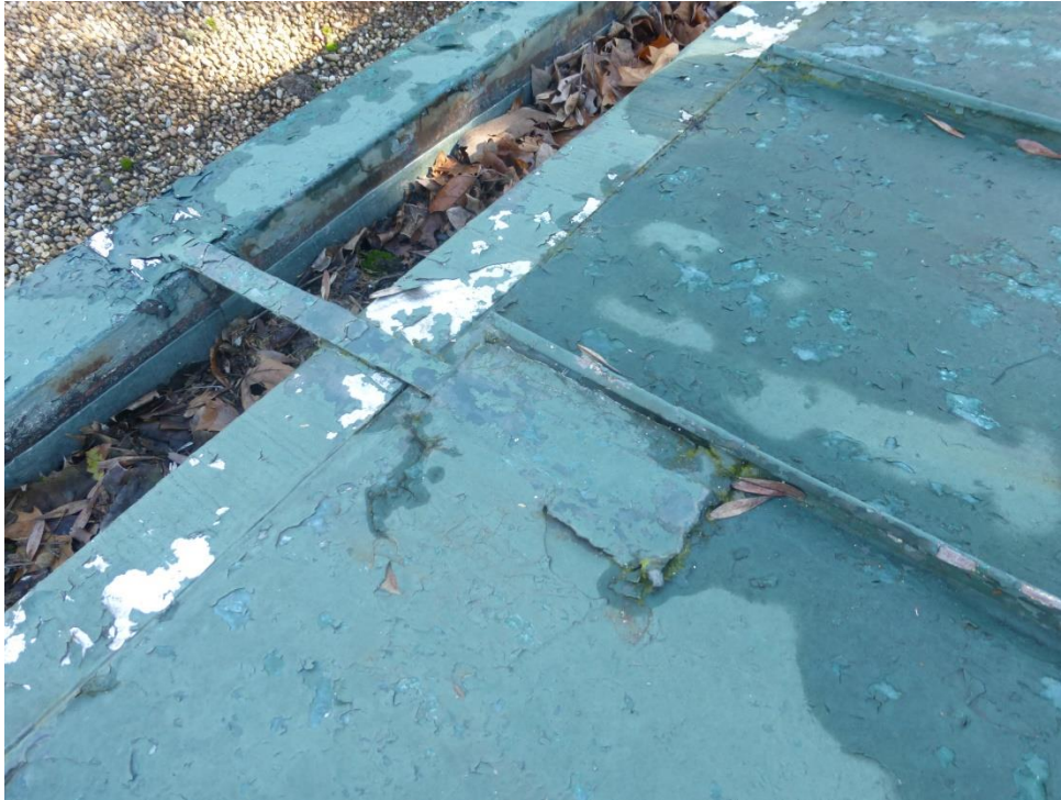
Eave Gutter Support Strap Attachment to Standing Seam Roofing
