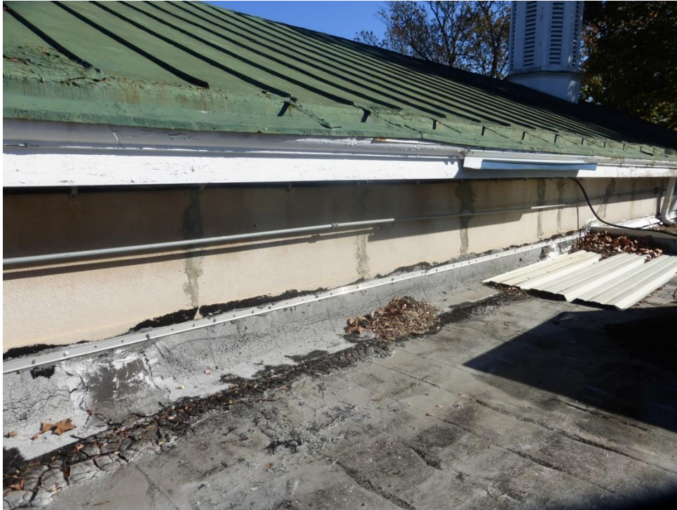
Repairs to Stucco Band below Double Sloped Standing Seam Roof
