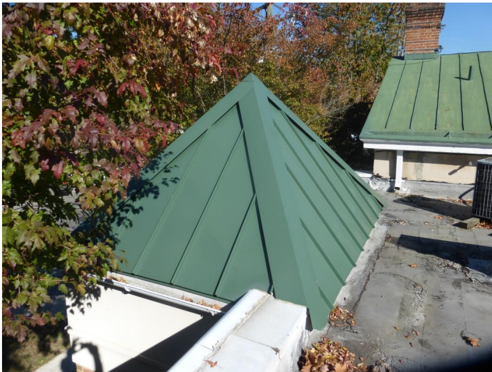
Steep Sloped Standing Seam Hip Roof
