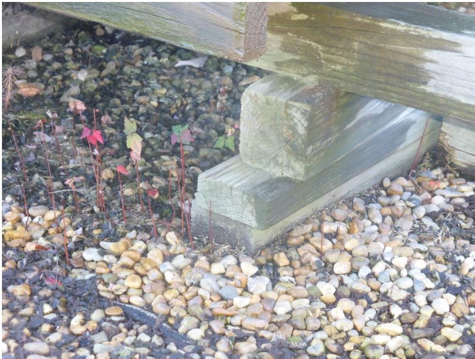
4 x 4 Lumber Supports for HVAC Unit- Notice how they are embedded into the membrane.
