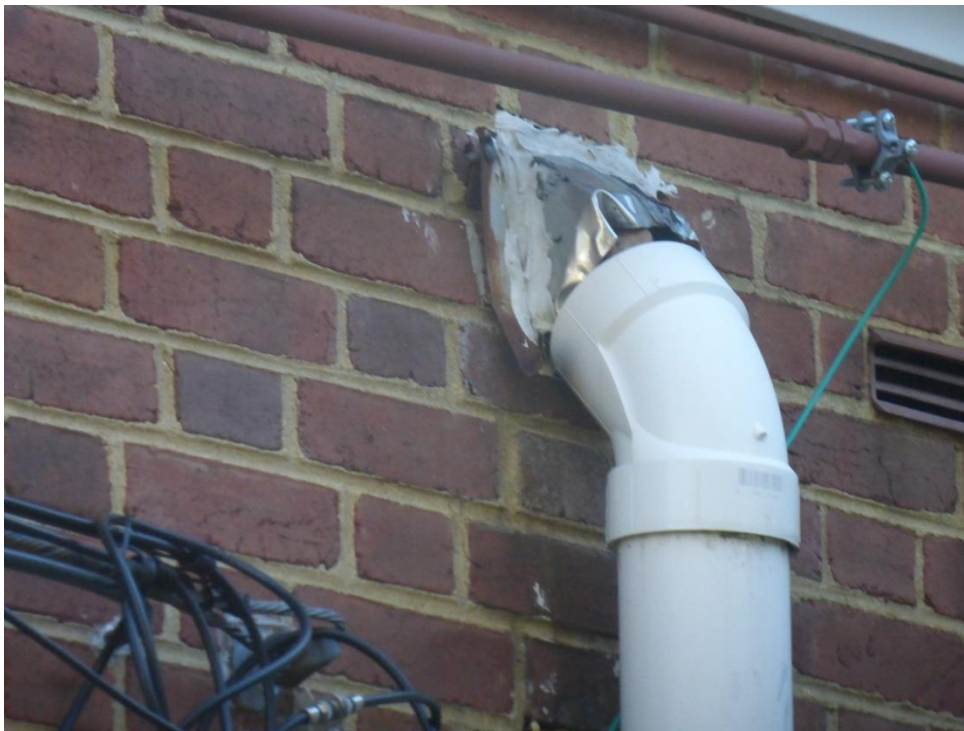
Very Poor Through Wall Scupper Repair
