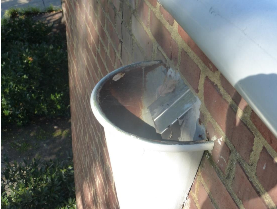
Typical Through Wall Scupper and Conductor Head
