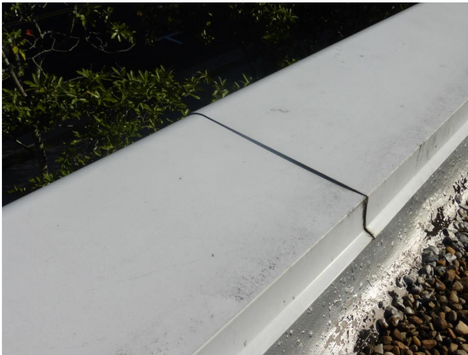
Open End Lap Joints in Parapet Wall Coping
