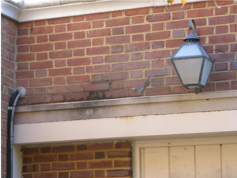
Water Infiltration into Masonry Wall
