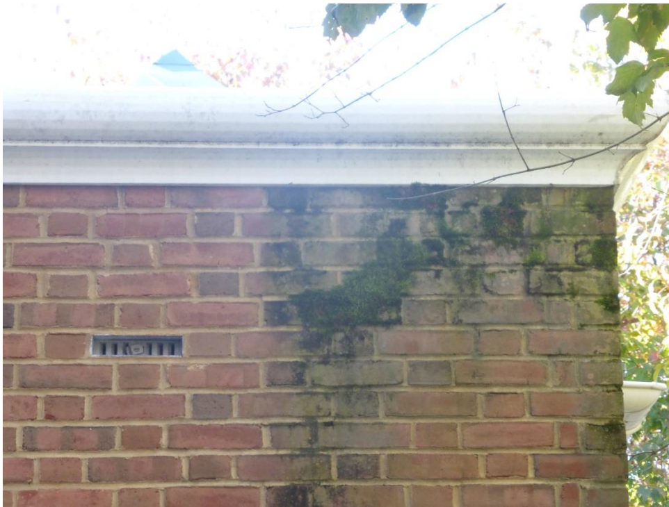
Water Infiltration into Masonry Wall
