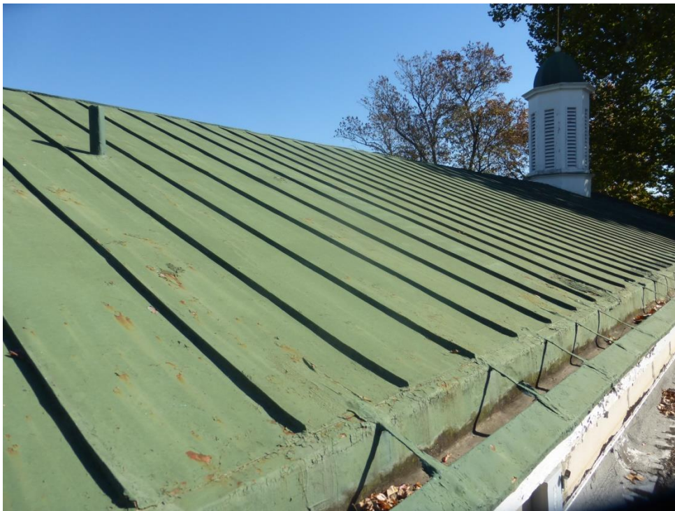
Double Sloped Standing Seam Roof (Tin Roofing)
