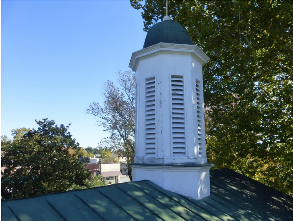
Cupola on Double Sloped Standing Seam Roofing
